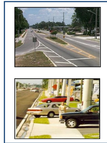
3: No Access Control
