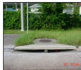
Curb Inlet with Manhole
