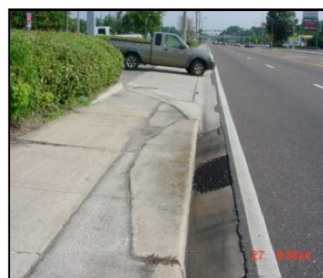
Curb Inlet without Manhole
